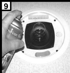
For a tile ceiling installation, the speaker is typically mounted to the tile and C-ring/rail assembly before the wiring is terminated (as was already described in step **2**). Once the wiring termination has been completed, place the speaker/tile/C-ring assembly on the ceiling grid.
