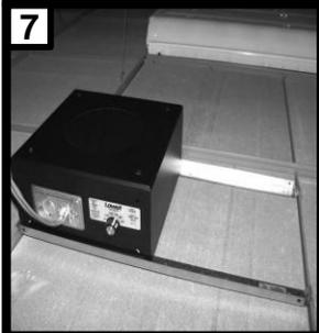
**7** Place the masking speaker with the bridge rails attached above the finished ceiling across the tile grid as shown.
