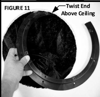
**Step-10:** Rest the ring and enclosure on the ceiling at the edge of the hole. Insert the four (4) 8-32 screws provided through the four (4) open holes in the lip of the enclosure into the four (4) threaded Tinnerman clips on the plastic trim ring. To make tightening the screws easier, spin the ring and enclosure so the screw you are inserting is at the center of the hole in the ceiling (shown in **Figure 14**).
