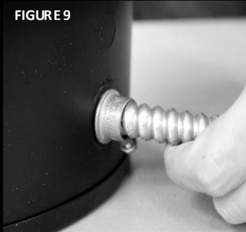
**Step-5:** If flexible conduit is required for the installation, install the proper flex conduit fitting in one of the 1/2"-3/4" conduit knockouts (shown in **Figure 9**).
